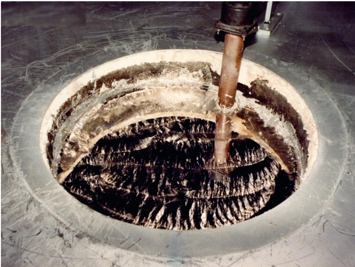
SIMPLE SKIMMING TEST DEMONSTRATES ALUMINUM SURFACE REACTION WITH PRODUCTS OF COMBUSTION. NOTE CLEAN, HIGHLY REFLECTIVE SURFACE IN ELECTRIC MELTING FURNACE ABOVE. PHOTO COURTESY SKS DIE CASTING & MACHINING, ALAMEDA, CALIF.
