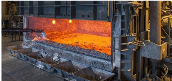
WET BATH REVERBATORY CENTRAL MELTING FURNACE
